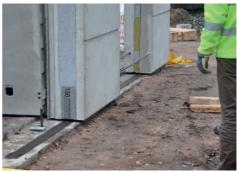
The CC-Window sealer is used for both vertical and horizontal installations. Attach the sealer with a small nail to the Styrofoam when sealing the construction elements in a vertical position. Align the CC-Window sealer and then place the construction element on top of the product. This gives you a fast, safe and time effective installation. The formula of CC-Window sealer makes it impossible for any mold to grow inside the product, in the rare coincident that any moister gets inside.
